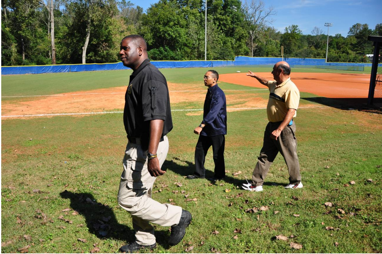
CEO Ellis, Public Safety Director Miller and Marist High School Facilities Director Art Diaz inspect water damage at ball field
